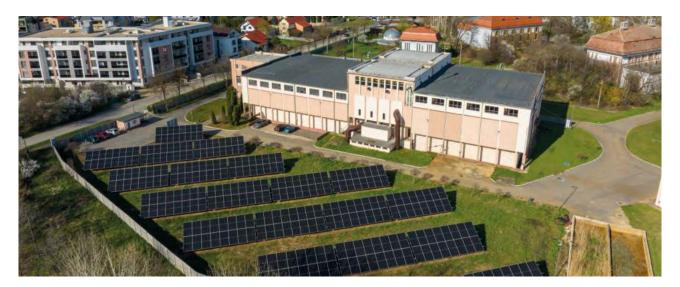
The photovoltaic plant at the WWTP produced last year 1.43 GWh and generated a reduction of 650 tons of carbon emissions, equivalent to planting 890 trees, while the one at the treatment plant Urseni produced 305 MWh.
